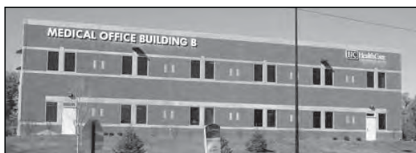
Alton Memorial Hospital's second and newest medical office building, which welcomes the public to its open house on Feb. 9, houses a consolidated, expanded Oncology Services department.
